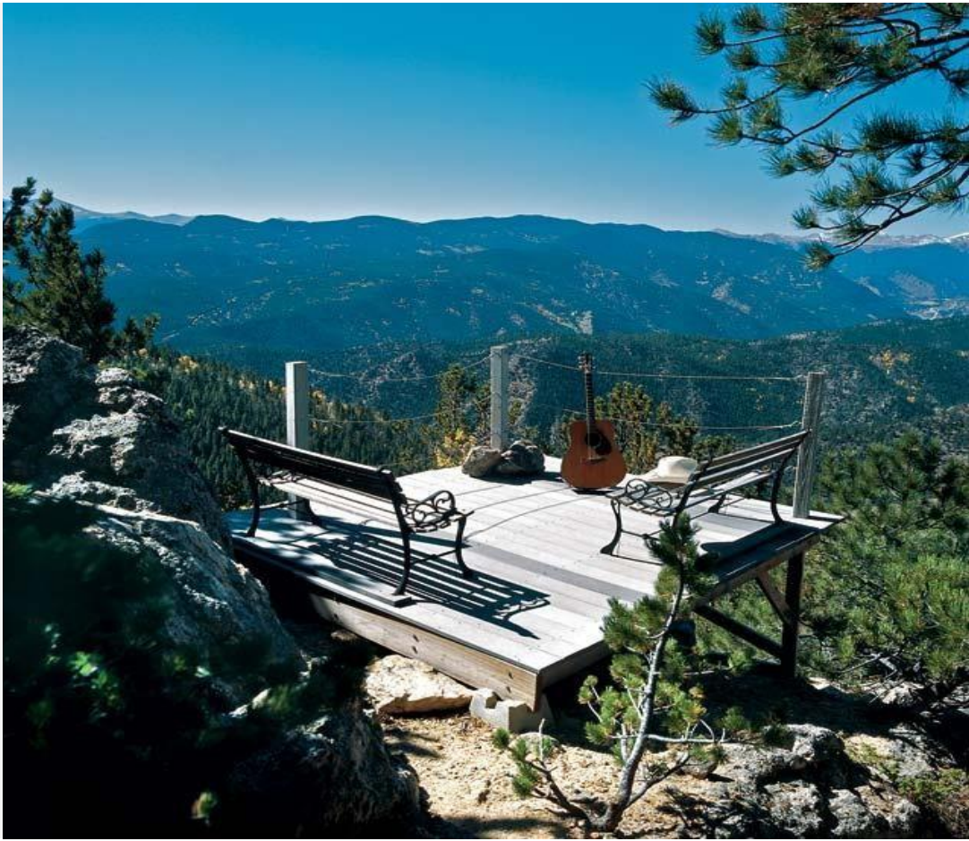
This 100-square-foot composite deck sits high above the mountains and provides the perfect vantage point for listening to area wildlife. Metal cables between the corner posts provide safety without obstructing views. Credit: James Ray Spahn photo
